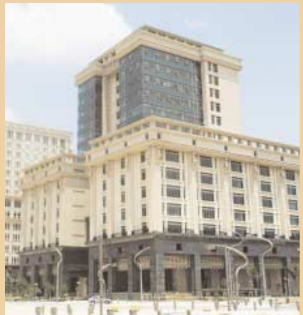
The National Registration Department Building in Putrajaya - Data Centre / Bangunan Jabatan Pendaftaran Negara di Putrajaya - Pusat Maklumat
