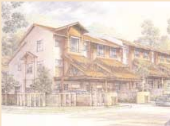
Sunway Bukit Gambier – A 23-acre development in a prime, upmarket location in Penang Island scheduled to be launched in mid 2005.
